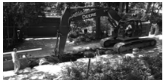
A new storm sewer was put under Campbell Street in 2020.
